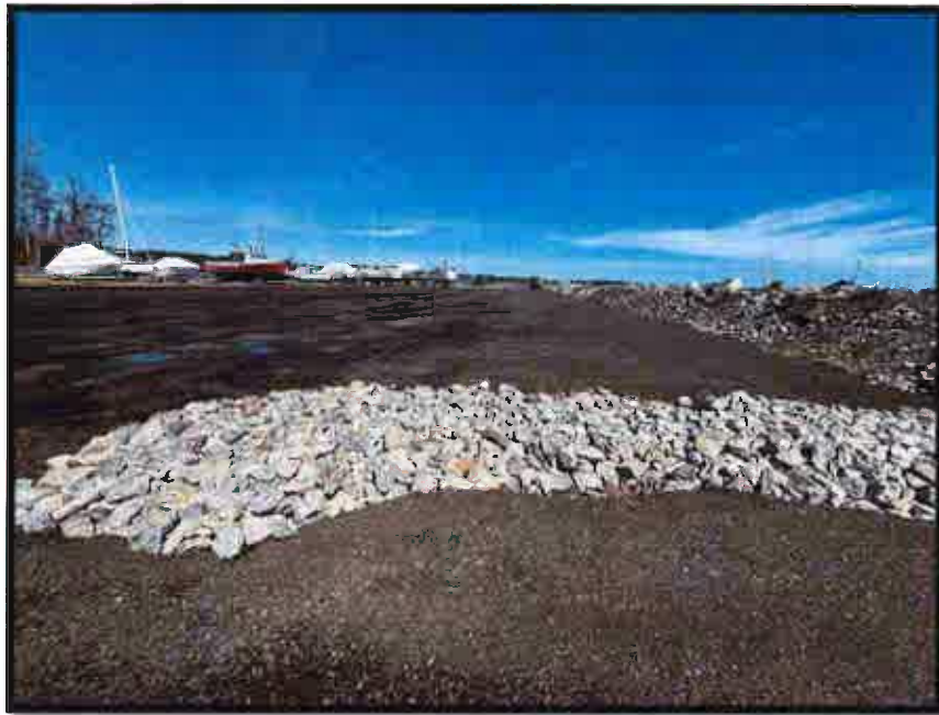
Rye Harbor Regrading and Parking Lot Drain Repair
